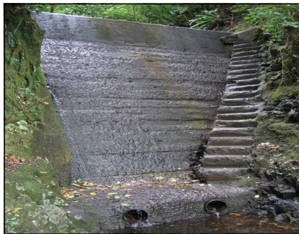
Figure 2. A reservoir built on a stream to supply villagers with water. These were typically built long before the municipal distribution system reached a village. Residents continue to rely upon them as a source of drinking water.
